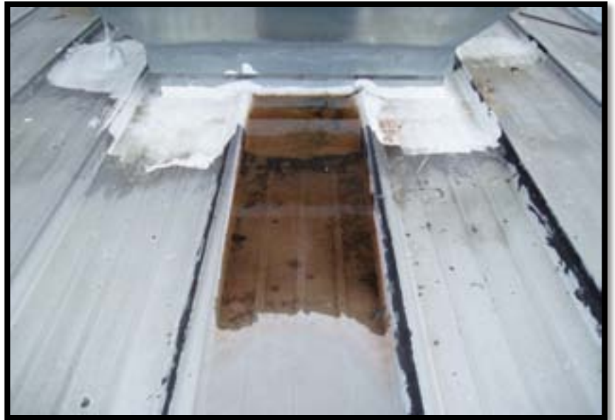
Improper assembly of curbs resulting in ponding water
