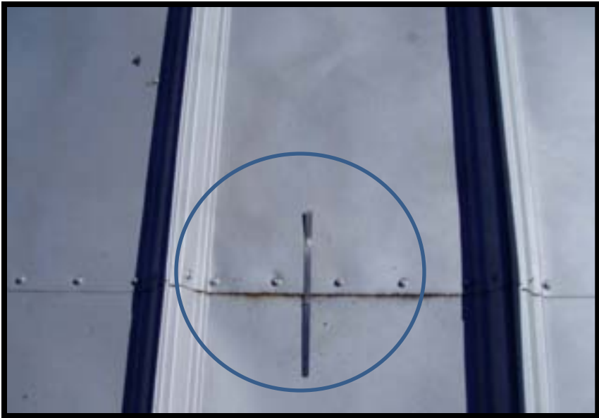
Missing panel lap mastic seal on a low slope roof will most likely leak
