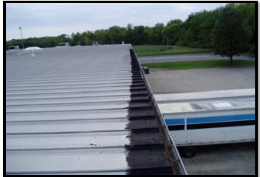
Improper use of carbon laden black mastic will oxidize metal panels in the presence of moisture
