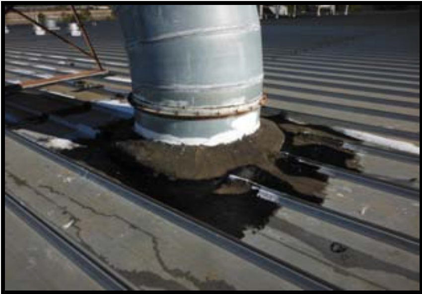
Improper use of carbon laden black mastic will oxidize metal panels in the presence of moisture
