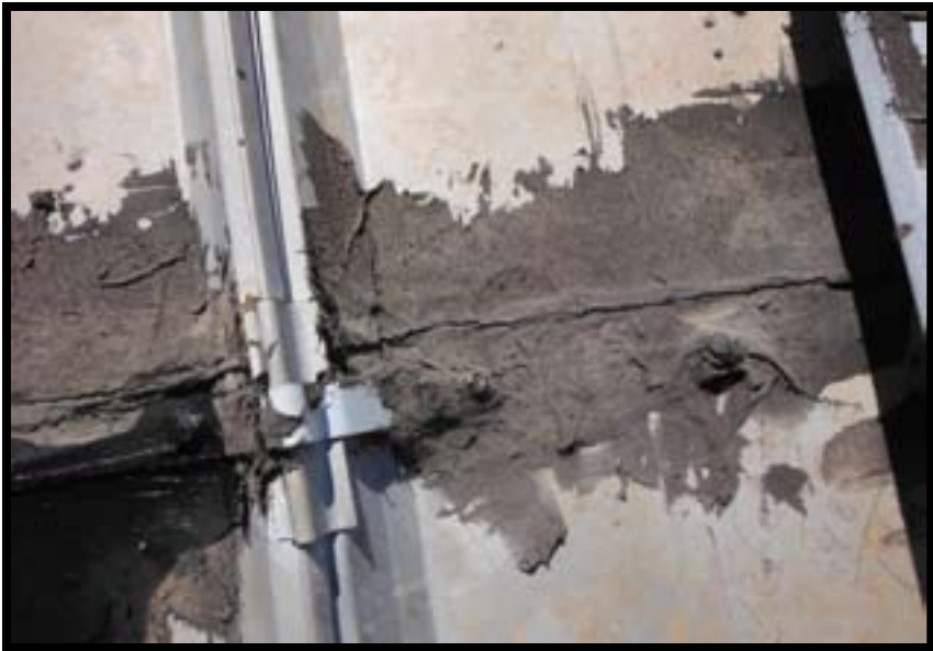
Improper use of carbon laden black mastic will oxidize metal panels in the presence of moisture
