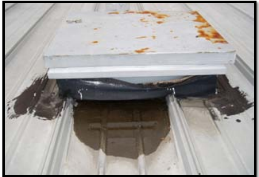
Improper assembly of curbs resulting in ponding water
