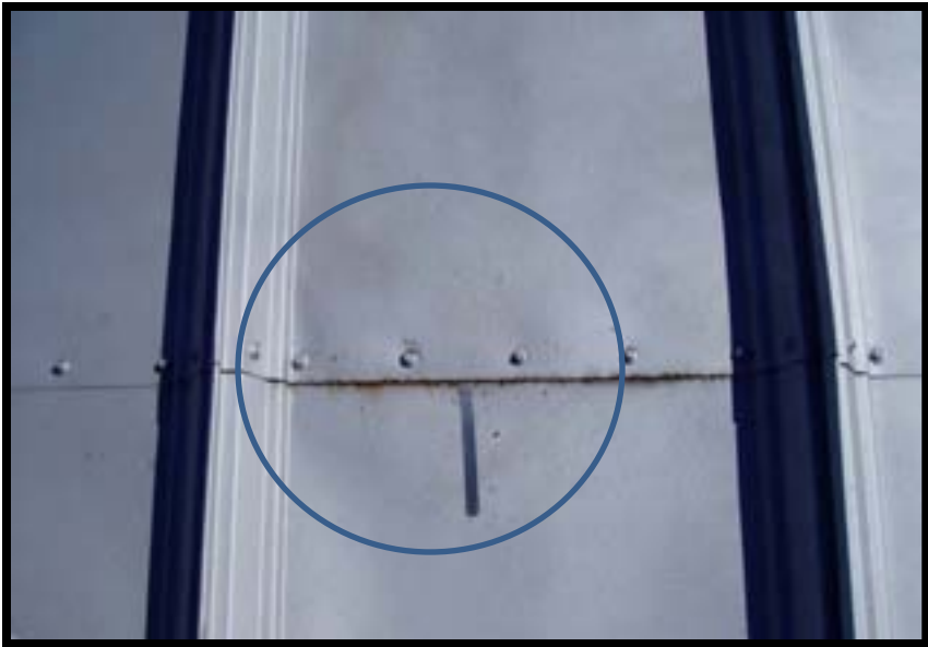
Missing panel lap mastic seal on a low slope roof will most likely leak
