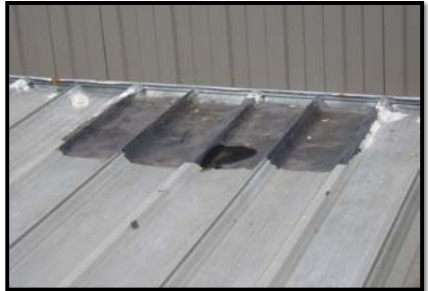
Improper use of carbon laden black mastic will oxidize metal panels in the presence of moisture
