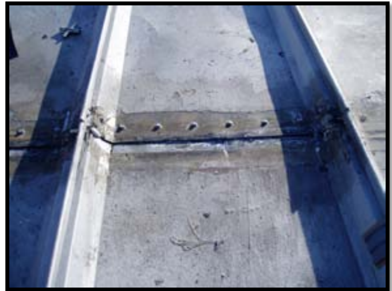
#4 Inject tube grade butyl at ribs, reassemble and install 1 st oversize fasteners
