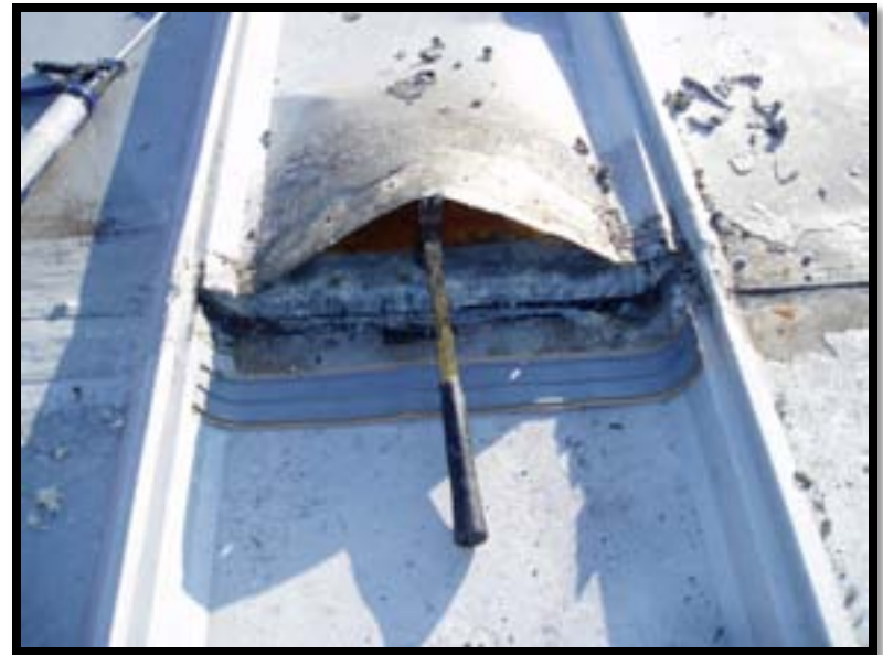
#2 Separate panels and clean internal surfaces
