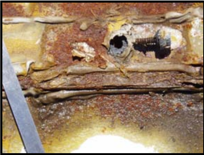
Improper external sealing material application to SSR system results in ponding water, more leaks and panel deterioration
