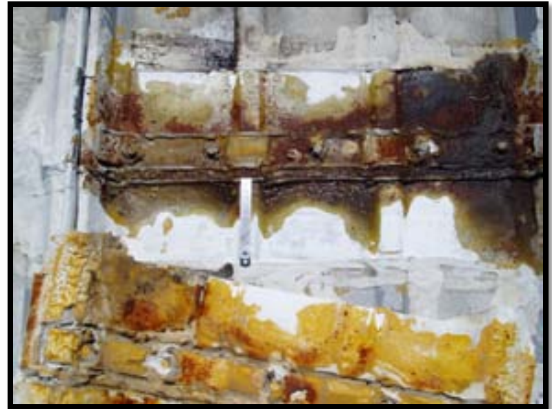
Improper external sealing material application to SSR system results in ponding water, more leaks and panel deterioration
