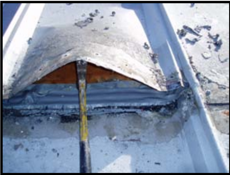
#3 Install triple “elastomeric-butyl” bead mastic between panels
