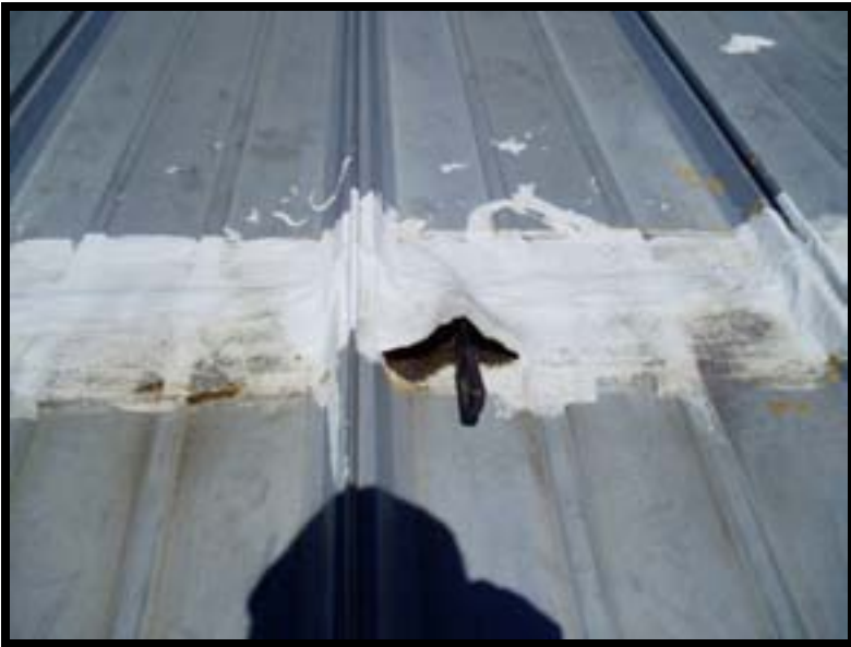
Improper external sealing material application to SSR system results in ponding water, more leaks and panel deterioration
