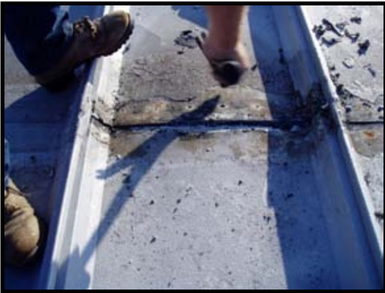
#1 Remove external material applications and fasteners
