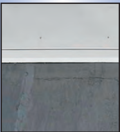
After - Reinforced open seams by using a three-course flashing repair system including a fibrated asphalt emulsion coating.
