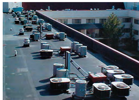
The huge amount of equipment placed on this EPDM roof will require careful monitoring by maintenance personnel.
